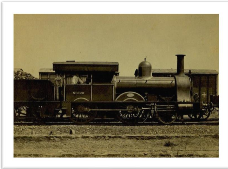
Source: Infrastructural Development in East Indian Railway
